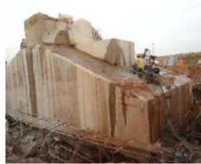
Fig. 5.27 Diamond Wire Sawing job for bridge pier
