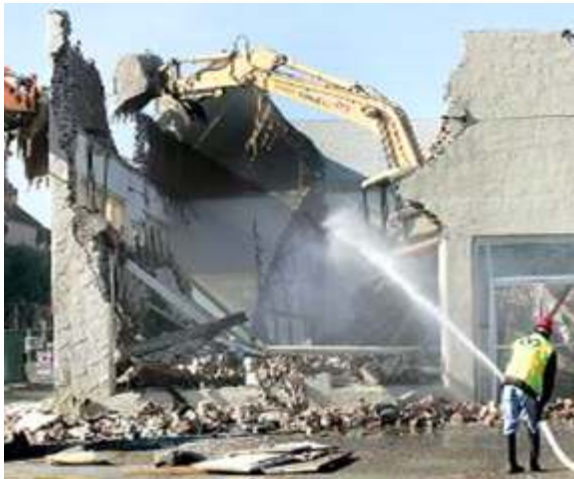
Fig. 2.6 (a) Dust control during deconstruction
