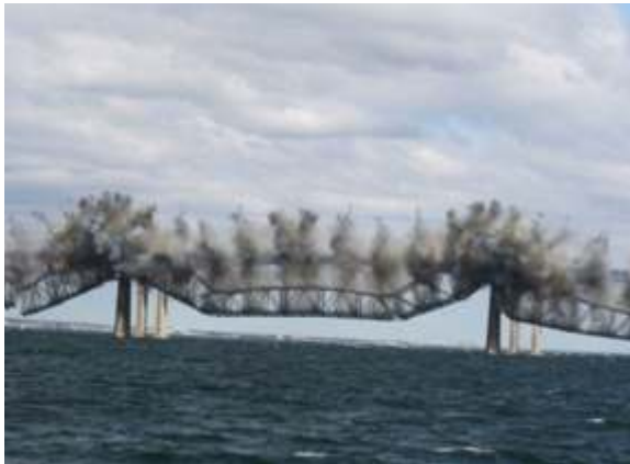
Fig. 5.42 Implosion of steel bridge in USA
