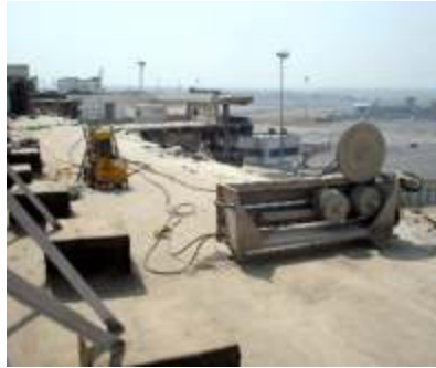
Fig. 5.26 Diamond Wire Sawing job in airport
