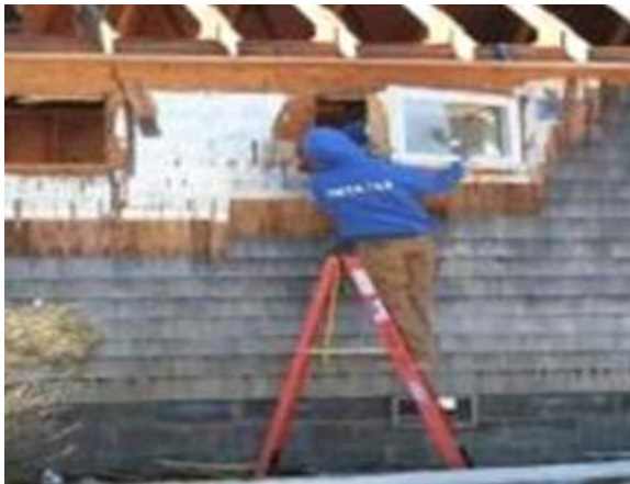
Fig. 4.1 (a) Non-structural deconstruction – Window
