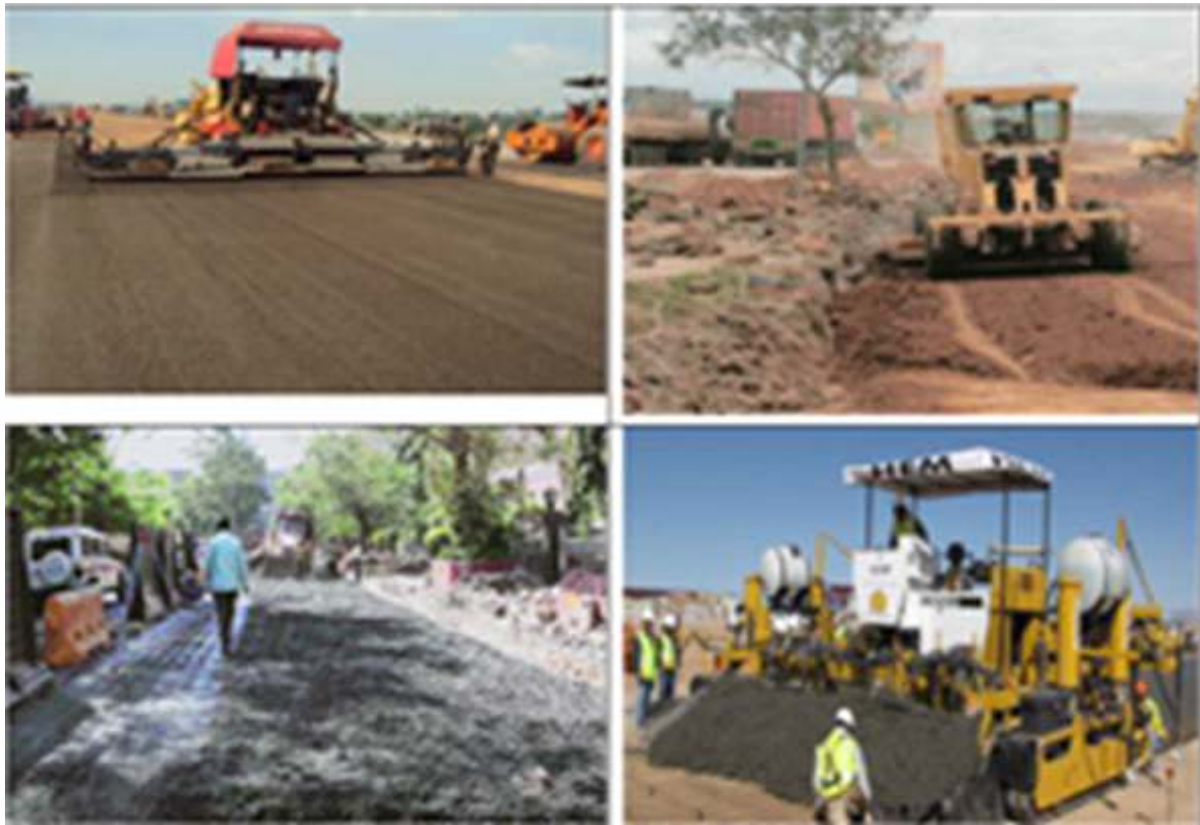
Fig. 5 Pilot road project by DDA using processed C&D Waste
