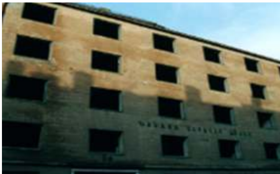
Fig. 4.1 (b) Building is fully stripped and prepared for demolition
