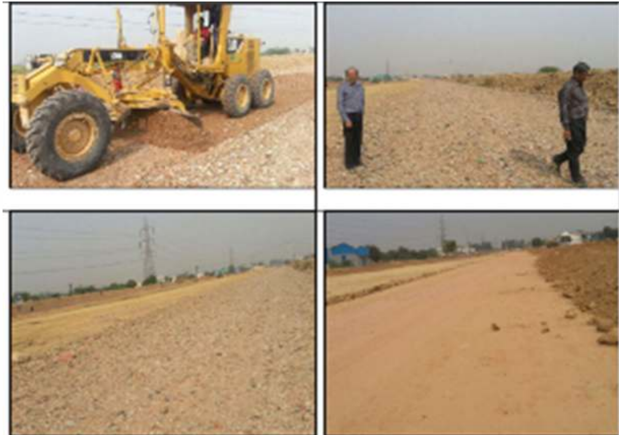
Fig. 4 Construction of access roads to the plant using recycled aggregates
