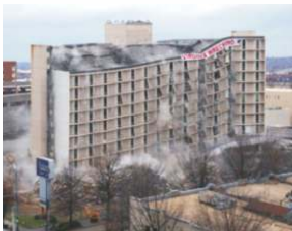
Fig. 5.40 Implosion of building
