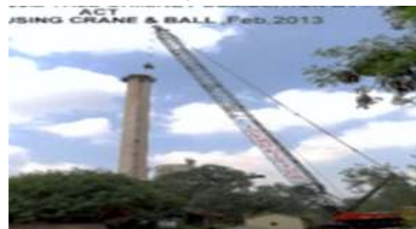
Fig. 5.34 Wrecking ball for chimney demolition
