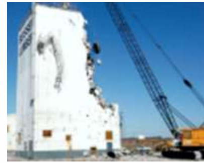
Fig. 5.32 Wrecking ball for building demolition
