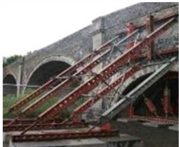
Fig. 3.7 Temporary supports – shoring and strutting
