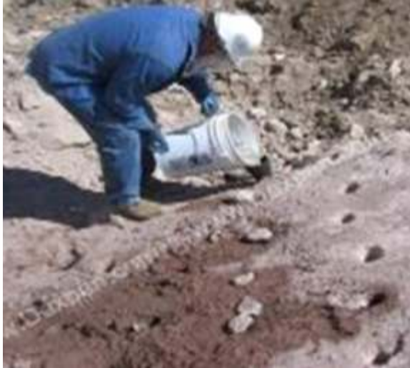
Fig. 4.3a, 4.3b, 4.3c, 4.3d Silent deconstruction chemical
