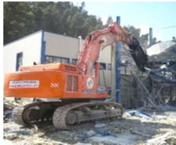
Fig. 5.17, 5.18, 5.19 and 5.20: Steel Scrap Shear mounted on Hydraulic Excavator on demolition, scrap handling and ship building jobs
