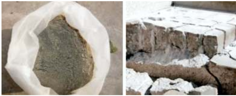
Fig. 5.30 and 5.31 Typical cracking using expansive agent
