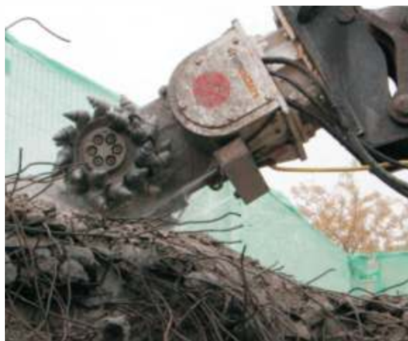
Fig. 5.21 and 5.22 Rotary Drum Cutters on RCC demolition job
