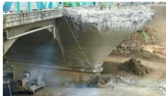
Fig. 5.29 Diamond Track Wire Saw on large bridge pier demolition
