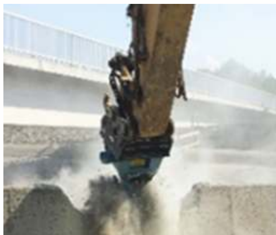
Fig. 5.21 and 5.22 Rotary Drum Cutters on RCC demolition job
