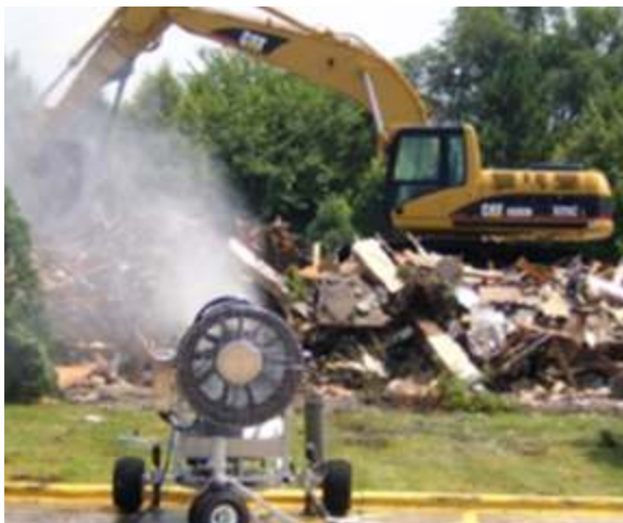
Fig. 2.6 (b) Dust control during deconstruction
