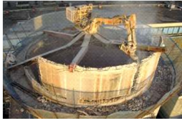
Fig. 5.48 and 5.49 Specialised drive lines chimney breaker
